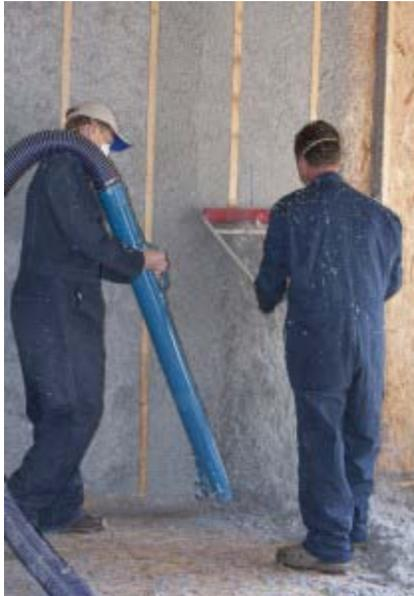
outside air is not able to penetrate. Creating a quality seal is the easiest way to reduce home energy usage and lower your monthly utility bill\*. Cellulose insulation is durable and treated to be fire retardant, insect resistant, and protected against mold and mildew. It is also renowned for its sound deadening qualities.
