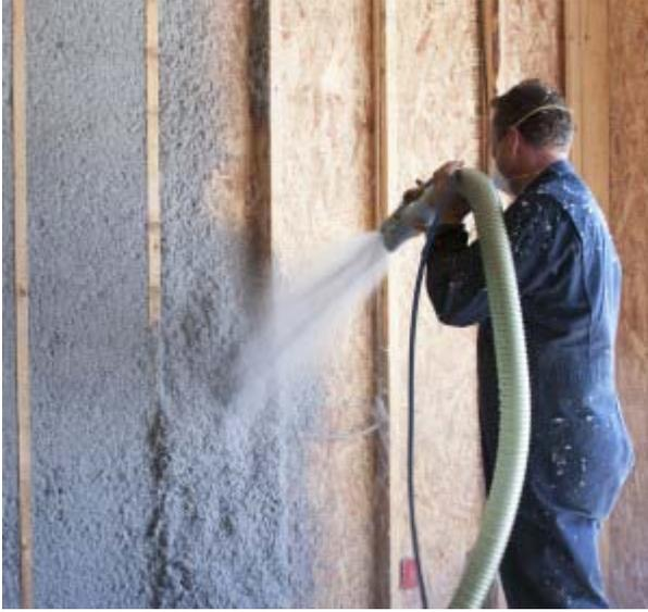
Nu-Wool Premium Cellulose Insulation is sprayed directly into the wall cavity.
