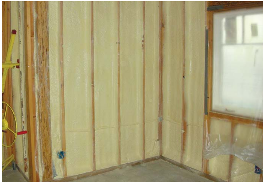
Right: To save costs, some builders use a hybrid insulation system called flash and batt where 1 in. of closed cell spray foam is applied to the wall first, and then a standard fiberglass batt is installed over the spray foam.
