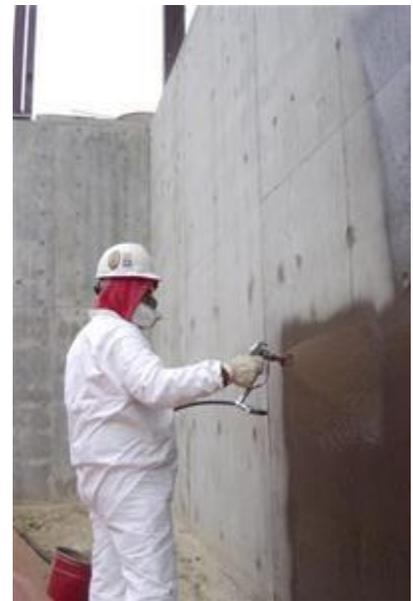
Of course the depth of the foundation wall and the use of the interior space will also determine the choice of methods. A 36-inch frost wall for an unheated crawlspace built on well-drained soil and employing a gravity drain is a good candidate for damp-proofing. The house next door with a 10-foot-high foundation wall and a finished basement might opt for a fully waterproofed foundation wall system
